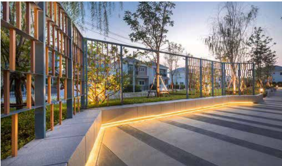
Pre cast concrete planters with lighting strip
